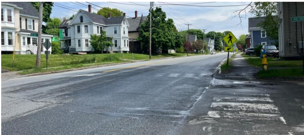
Figure 23 – Crosswalk at Holyoke Street across North Main Street
