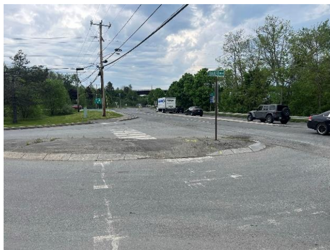
Figure 27 – Pedestrian crossing at I-395 Exit 4 Westbound Ramp encroaching on signalized pedestrian crosswalk
