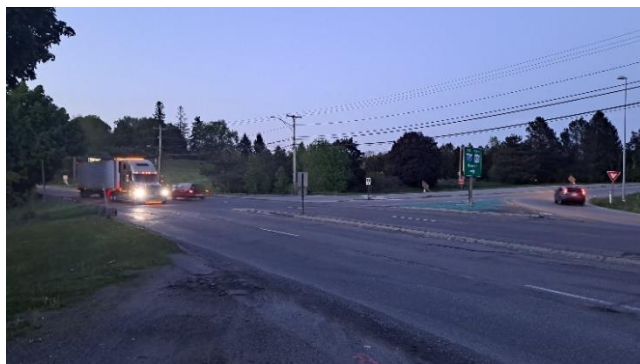
Figure 25 – Low-light conditions at I-395 Exit 4 Westbound Ramp intersection
