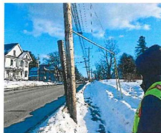
Image: 2 Utility Poles in pedestrian
