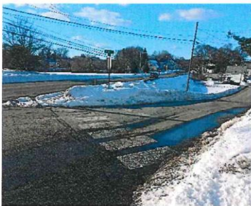
Image: 1 Parker – Wilson Intersection facilities along Wilson Street.
