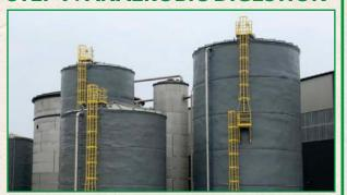
The watery stream of organic wastes, like food leftovers, flow into the anaerobic digester. Like a stomach, this digests the organics into a renewable natural gas, leaving the water clean. The clean water is recycled in a closed loop back into the system. The renewable gas is used to power Coastal, offsetting fossil fuels. In the future, it could also be used locally as a natural gas substitute to lower our community's carbon footprint.
